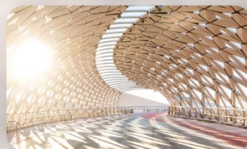
Atyrau Bridge Astana
